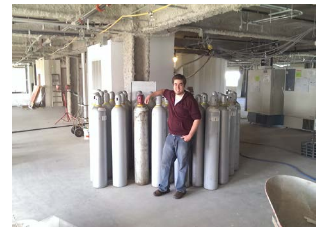
Team member Joseph Roberts stands next to the 48 CO2 tanks that had to be carried up four flights of stairs in the Holy Cross building. Each weigh approximately 200 pounds, and are vital to the operation of the ultra-cold freezers.
